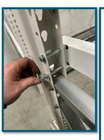
Note: Mallet may be used in this process to seat hardware in place.
